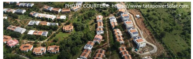
5.25 kW Solar Roof Top Power System installed on 42 cottages of Suvidha (2017). The original idea to use rooftops for solar power generation was first mooted by Prof R Sankar in 2015.
